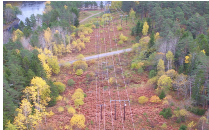
Power line inspection using drones
